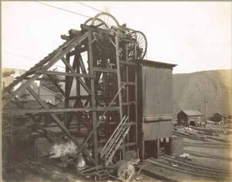
Coal Mines. Headframe of West Virginia mine. The large wheels at the top are for winding up the ropes. The structure is made of heavy timber. (1917)
