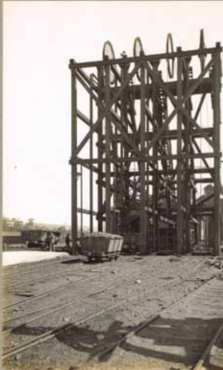
Coal Mines. Headframe of Coal mine, near Lanes, West Virginia. The large wheels at the top are for winding up the ropes. The structure is made of heavy timber. (1917)
