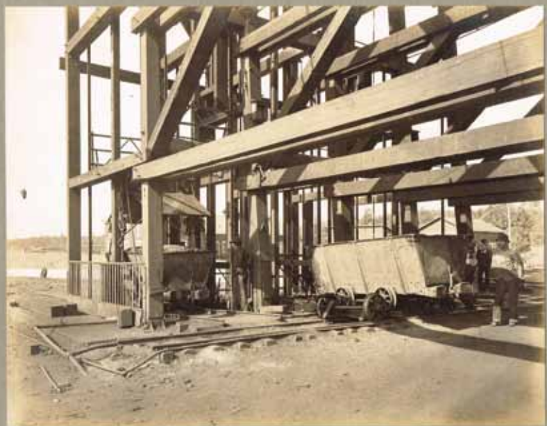
Coal Mines. Top of headframe. The large wheels at the top are for winding up the ropes. The structure is made of heavy timber. (1917)
